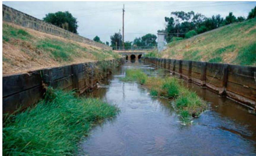
Looking down the drain towards the sampling site. Almost the entire length of the drain has wooden boards lining the sides. Photo: Dieter Tracey
