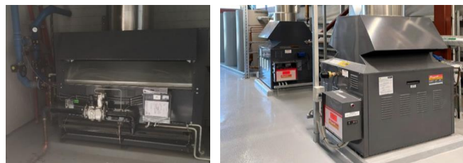
Figure 2: (Left) Reference photo of a commercial gas boiler system – utilised at the MLC & CCGS Aquatic Precinct in Western Australia. (Right) Gas boiler – reference image – courtesy of Raypak/Rheem.
