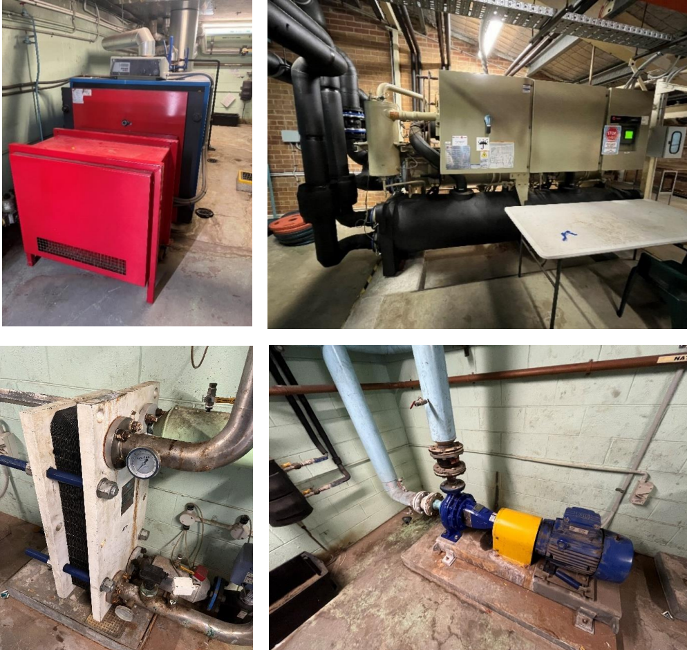
Figure 1: Reference images of the Bayswater Waves existing heating system infrastructure. (Top Left) The existing gas boiler. (Top Right) The existing chiller system. (Bottom Left) The existing heat exchanger infrastructure. (Bottom Right) The existing heating system circulation pump.
