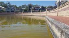
Vertical walls with steep underwater slopes present safety risk, Img: M P Rogers & Associates
