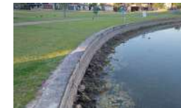
Retaining walls with rock armour limit areas for fringing vegetation, Img: google.com
