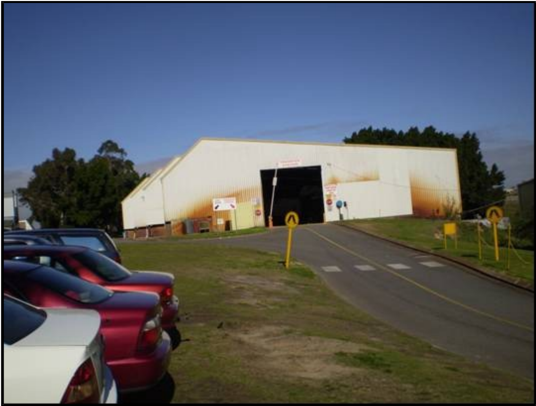
Figure 5- Solid waste disposal shed north side(entry)
