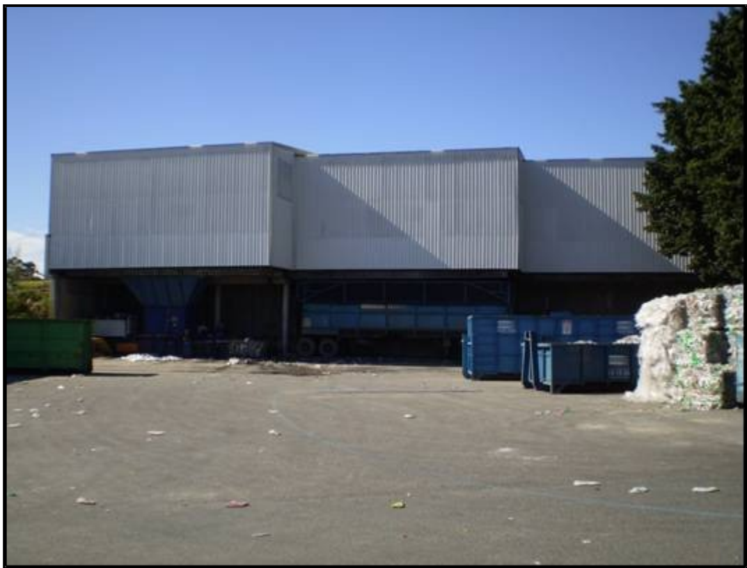
Figure 8 – Solid waste shed west side showing collection bins
