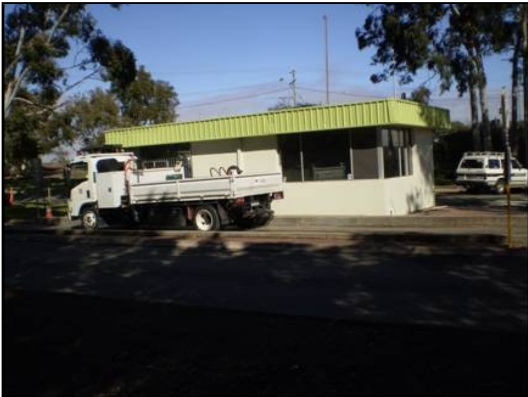
Figure 2 - Gatehouse exit eastern side
