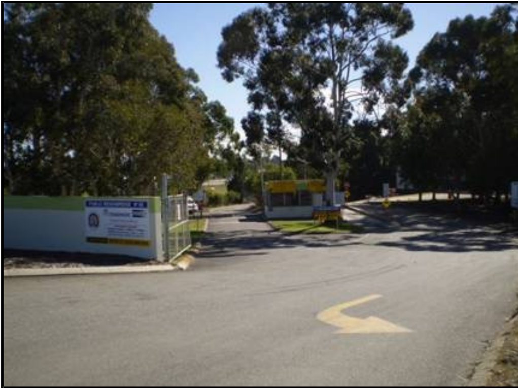
Figure 1 - Front view showing gatehouse and weighbridge
