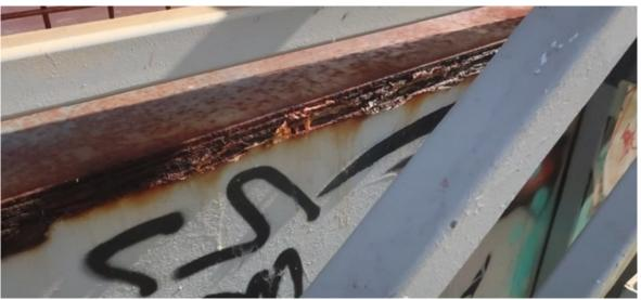
Significant corrosion at the edge of the eastern platform
