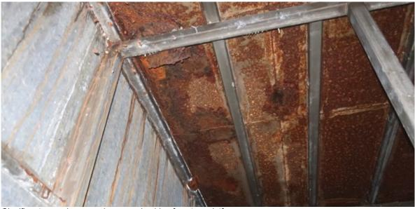
Significant corrosion occurring on underside of eastern platform
