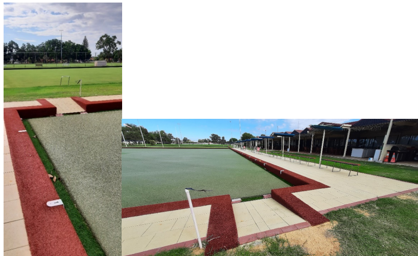
Image 1 and 2: Upgraded accessibility ramp at Morley Bowling Club.
