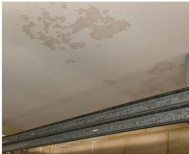
*Water damage in garage area on north-eastern side*
