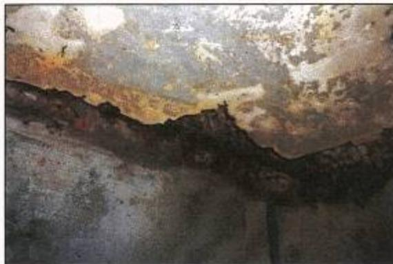
*Photo 3 The inspection revealed that inside the concrete structure was displaying cracking and delamination of the concrete to various degrees.*
