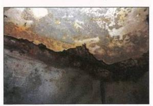
Photo 3 The inspection revealed that inside the concrete structure was displaying cracking and delamination of the concrete to various degrees.
