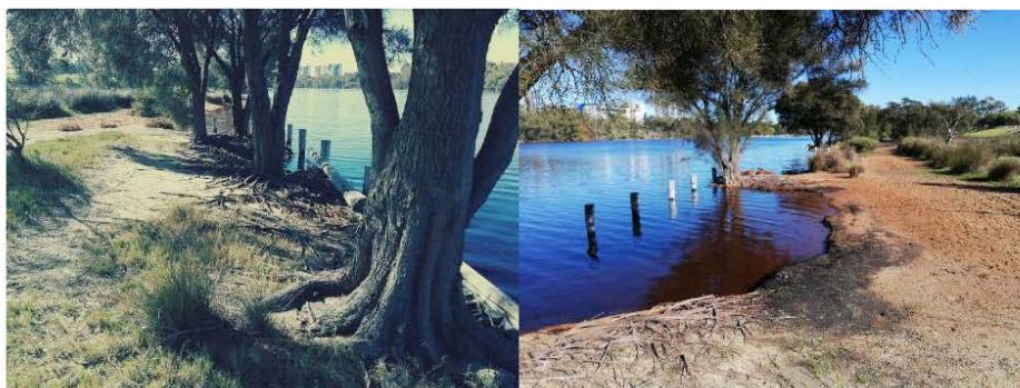
Figure 5.27 Undercut Trees at Maylands Timber Riverwalls
