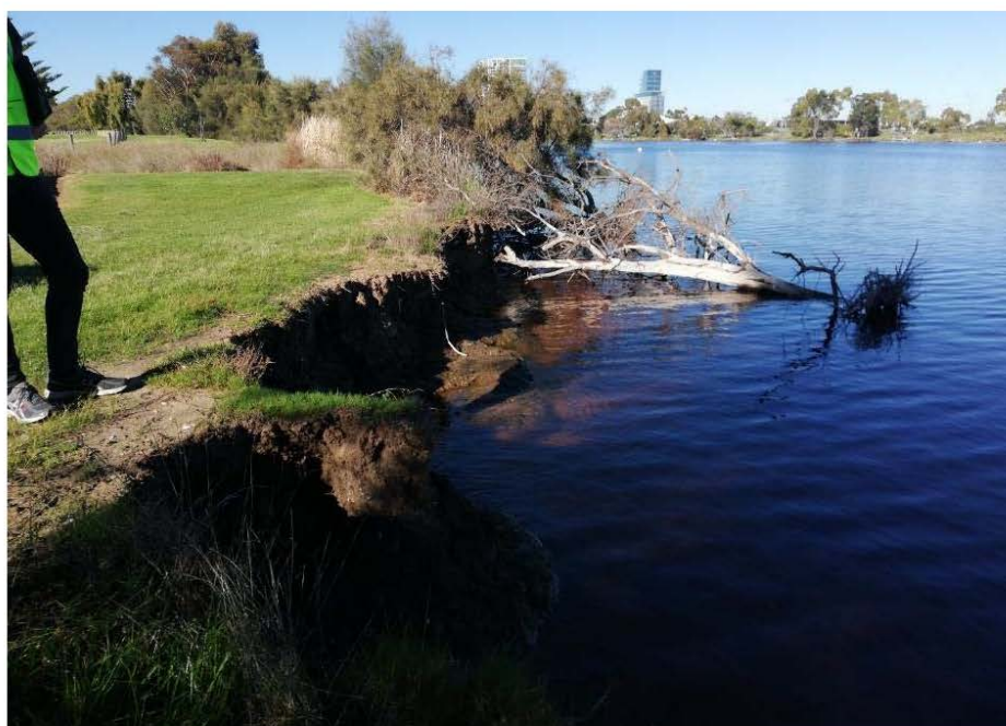
Figure 5.26 Erosion Scarp at the Maylands Peninsula Golf Course – Hole 5
