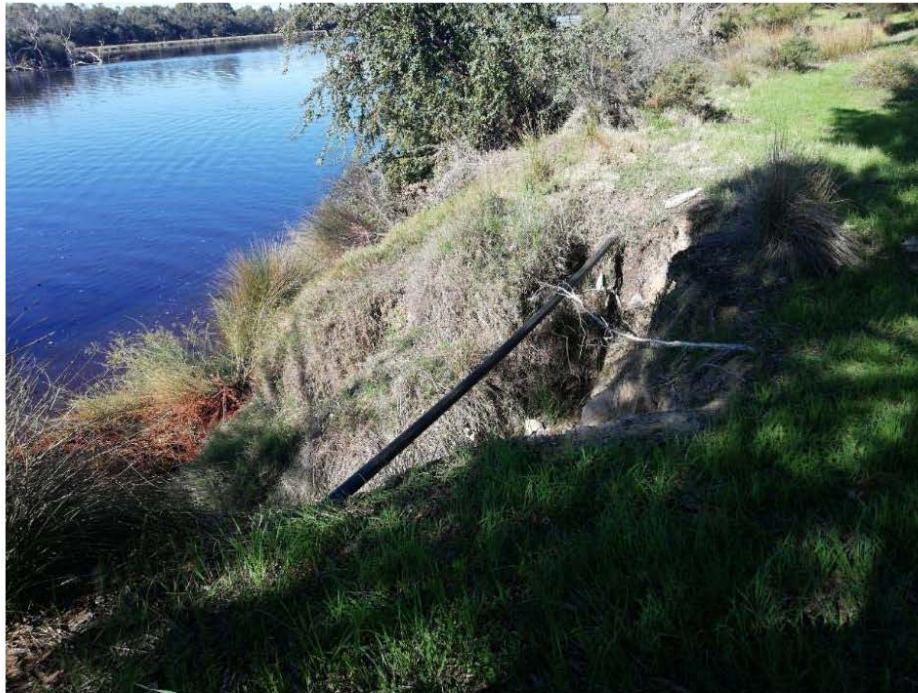
Figure 5.15 Eroded Riverbank & Exposed Water Corporation Asset
