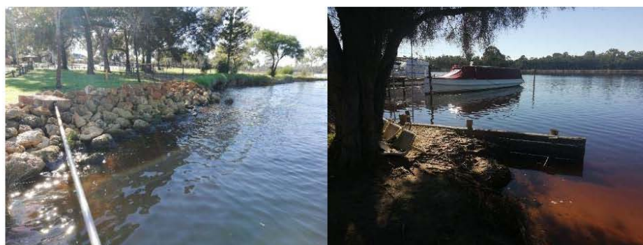
Figure 4.4 Built Shorelines, Left: Revetment, Right: Wall
