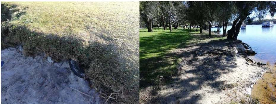
Figure 2.3 Uncontrolled Fill at Bardon Park (left) & Tranby Reserve (right)
