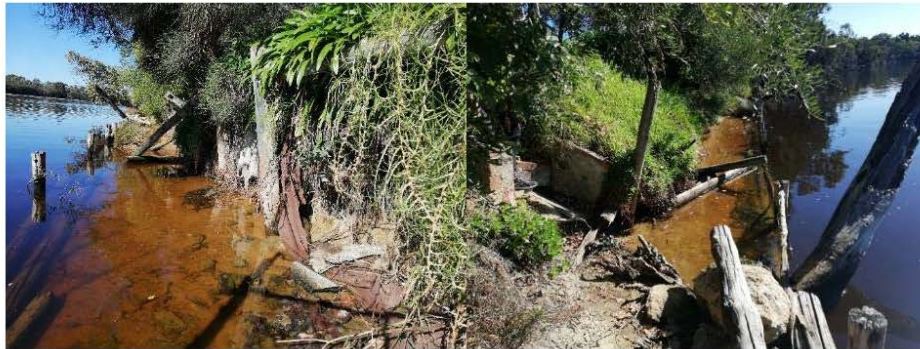
Figure 5.1 Failed Tranby House Reserve Timber Walling
