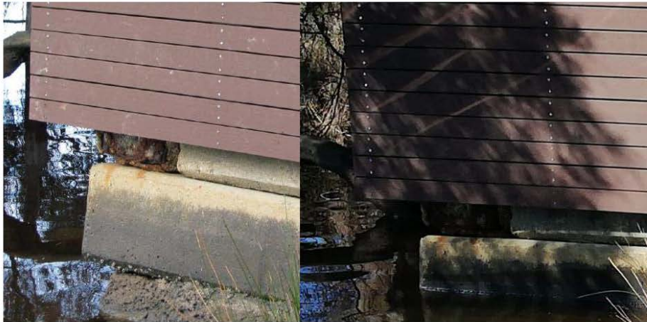
Figure 5.21 Abutment Beneath Gazebo, Left: 2013 (Cardno). Right: 2019
