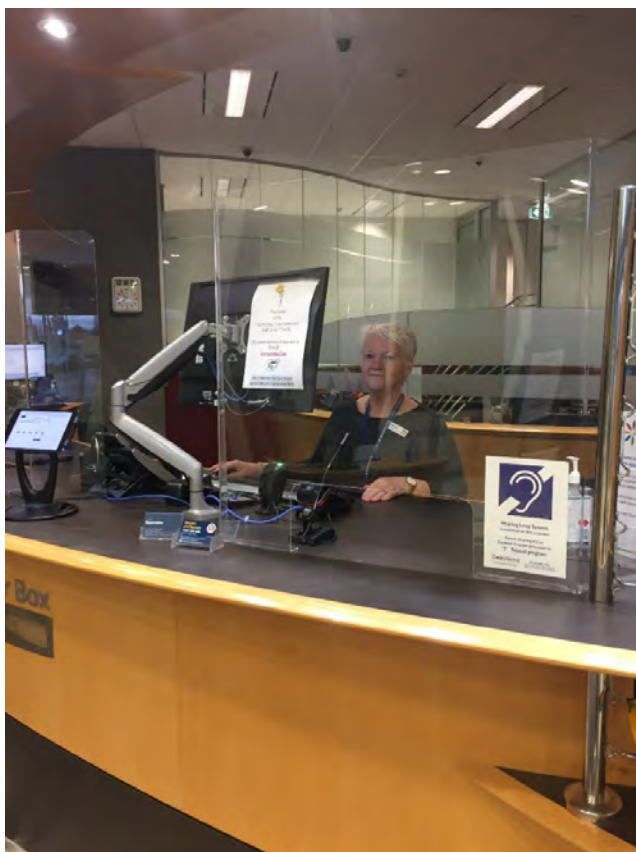
Image 8 ClearaSound Counter Hearing Loop System installed at the City of Bayswater Civic Centre, Customer Service counter, July 2020.
