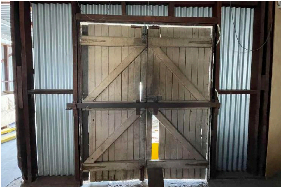
17 Storage Area Internal - ledge and braced timber paneled double doors
