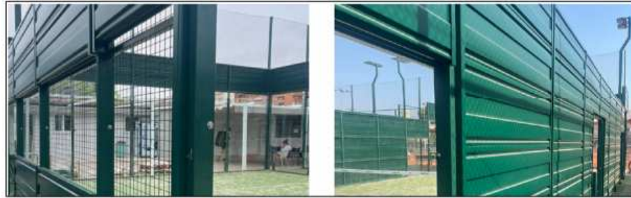
FIGURE G2 – PHOTO OF A PADEL COURT FITTED WITH THE ACOUSTIC PANELS
