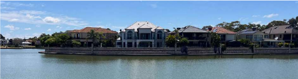
Continuous hard edge with steep slopes make it difficult for emergent plants to establish affecting water quality.
