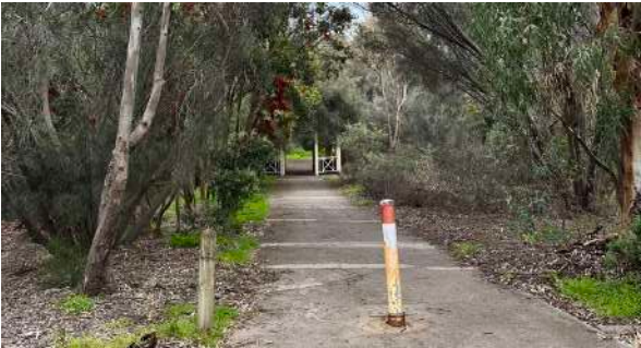
CPTED concerns from poor sightlines for pedestrians and no lighting.
