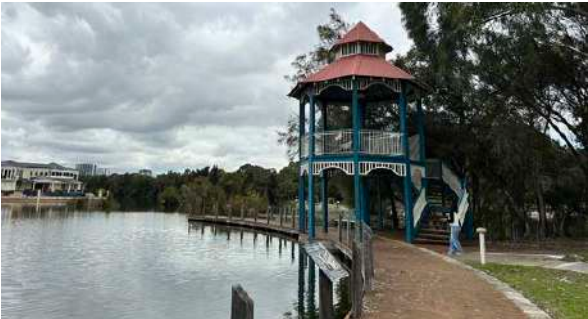
Gazebo provides view points across the lake, signage requires upgrading.
