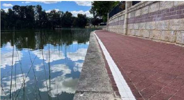
Drop off from path is a safety risk.
