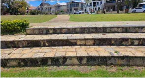
Terracing requires maintenance.
