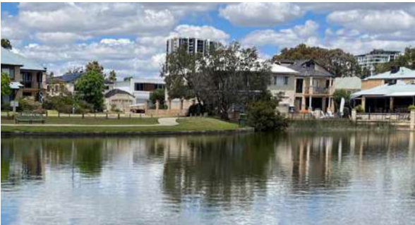
Hard wall edges limit emergent vegetation establishment contributing to poor water quality.
