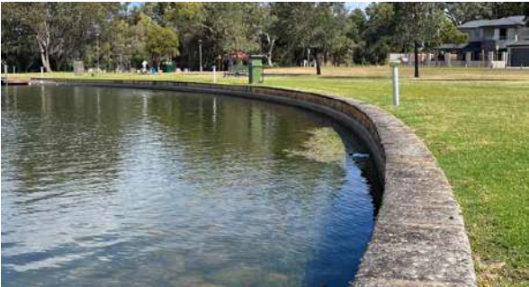
Limestone wall edges to lakes, drop off into water.
