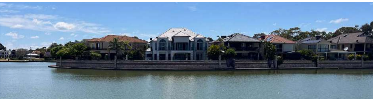
Continuous hard edge with steep slopes make it difficult for emergent plants to establish affecting water quality.
