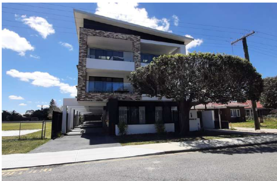
Figure 2 – Image of 1 Mangini Street
