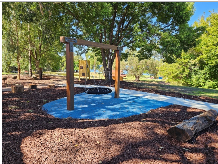
Image 3: Basket swing with new connecting concrete footpath with rubber soft fall
