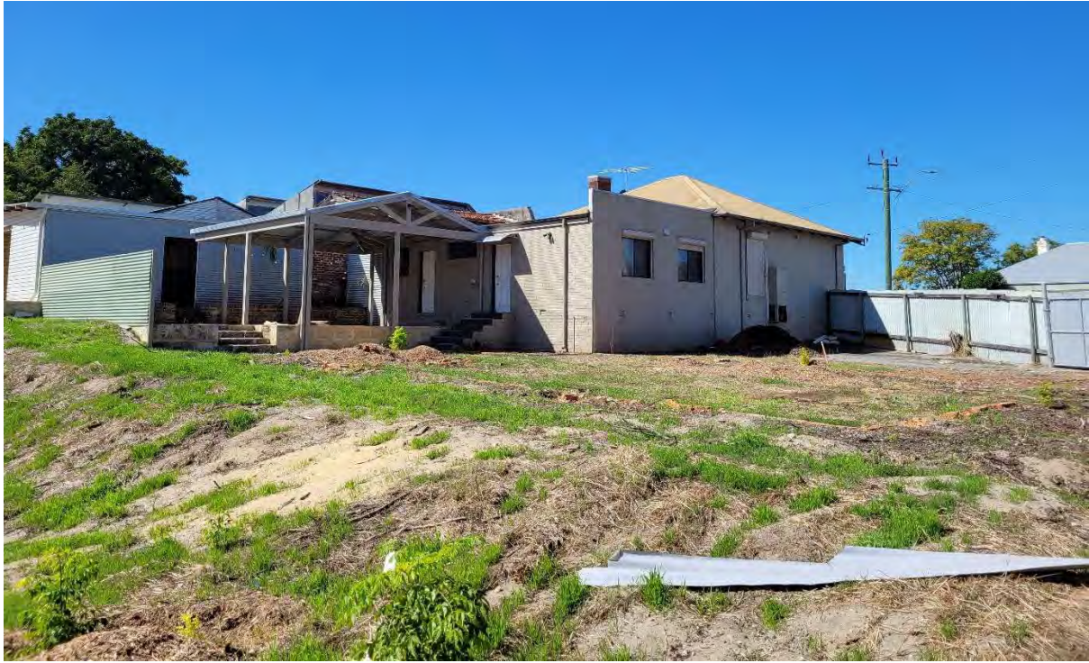
Photo 5: Existing buildings and site conditions, taken from Kenilworth Street.
