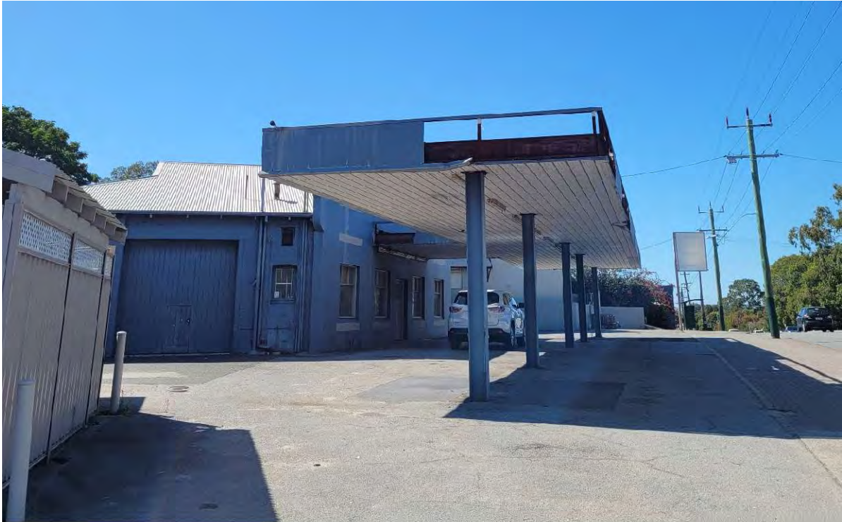
Photo 1: Looking east at the development site, along Guildford Road, noting existing buildings and canopy.
