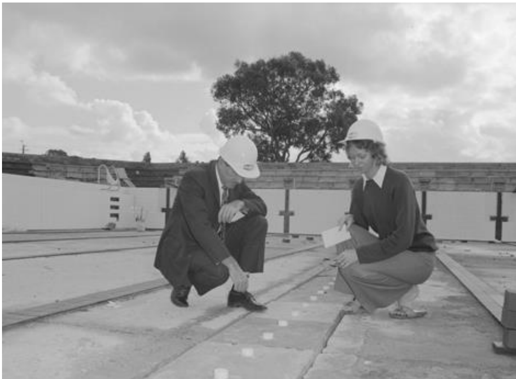
FIGURE 45 BAYSWATER SHIRE SWIMMING POOL CONSTRUCTION, 1971.
