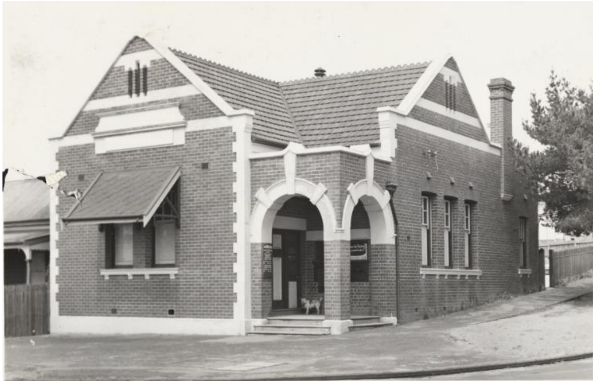
FIGURE 19 MAYLANDS POST OFFICE (BUILT 1910), 1942.
